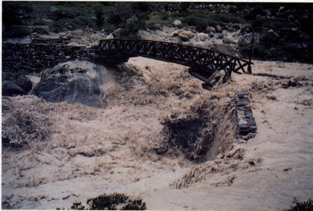
Plate 17 A small glacial lake outburst flood disrupting a bridge on the Dudh Kosi river, Central Nepal, July 1984 (photograph by J. Desloges).
